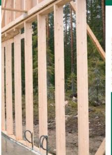
LamecoFrame® is a new type of glued frame pillar, LamecoFrame® is an ideal and dimensionally precise solution for all locations that require unbendable, durable and light supporting structure material, which has excellent glulam properties.
